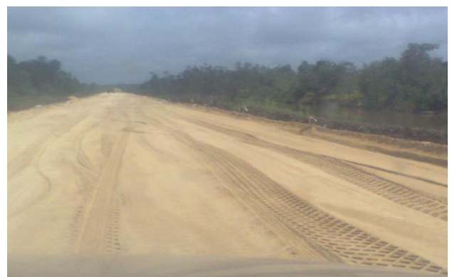
Figure 2: Cross-section of the Road (N 04°34'44.82", E 006°22'00.84")
