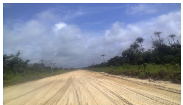
Figure 3: Cross-Section of the Road (N 04°36'35.52", E 006°20'46.74")
