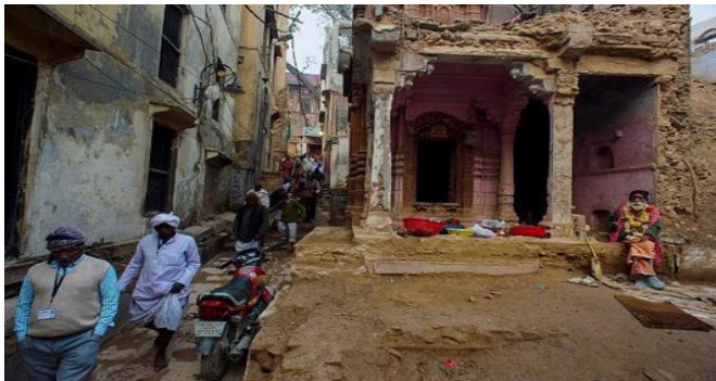
Figure 2: A sadhu sits in front of a damaged temple near Saraswati Phatak
